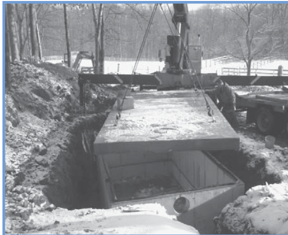
This rainwater collection system at Arcadia Farm in Yorktown channels roof runoff into an underground storage tank. While WAC helped correct soil erosion problems at this farm, this BMP allows the landowner to conserve and reuse the water on the farm. At the landowner's expense, the tank was connected to a pump and sprinkler system for irrigation during the summer months.
