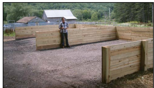
A Small Farm Planner inspects a newly constructed manure storage/composting facility. The gravel pad is located away from water courses and provides temporary manure containment until the manure is composted and spread according to the farm's Nutrient Management Plan.
