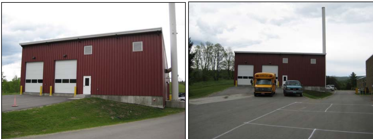
Figure 1 Typical School Woodchip Boiler Plant
