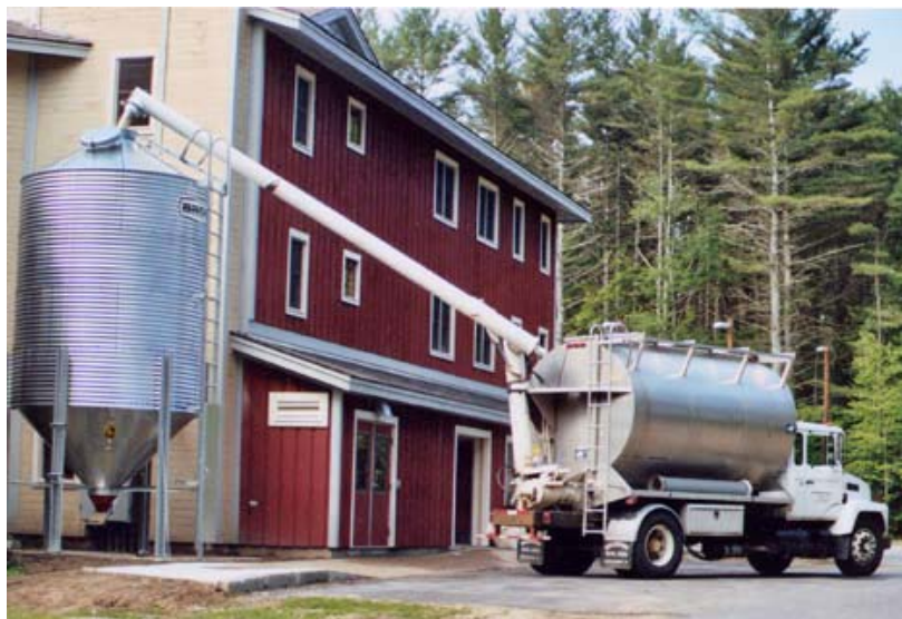
Figure 6 Typical pellet fuel storage and delivery 5
