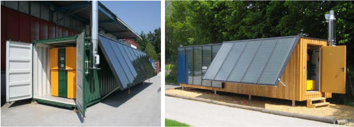
Figure 4 ACTbioenergy containerized pellet boiler system
