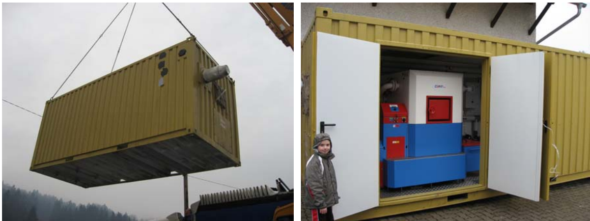
Figure 4 ACTbioenergy containerized pellet boiler system
