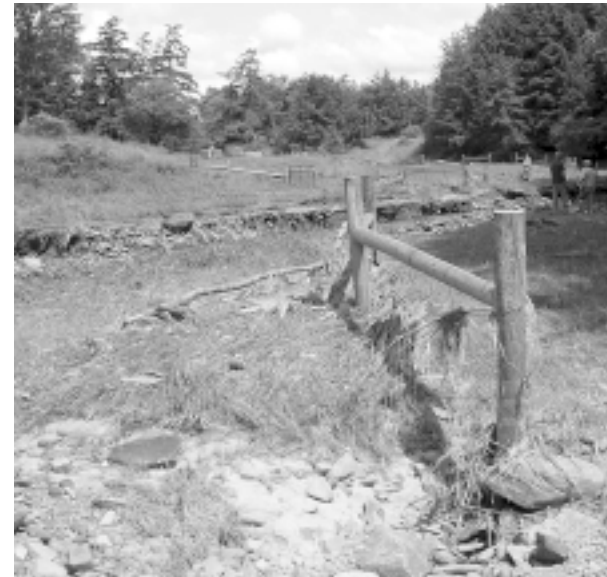
Stream buffers and bridges were taken by Third Brook at Healing Waters Farm in Walton.
