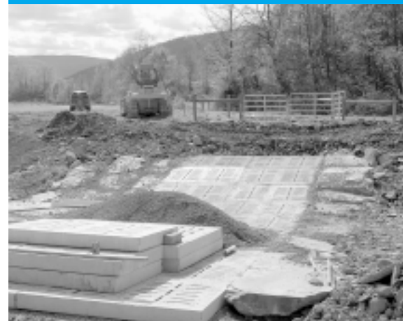
Cattle slats are relocated to a safer spot on Kerrs Creek after being dislodged by June’s floodwaters.
