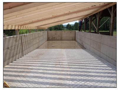
growing numbers and the site is just above a road ditch that would carry runoff to the nearby stream. A 35' x 40' roofed concrete barnyard was built that provides a small buckwall area for manure scraped out of the two exercise areas to be easily picked up and transported to the manure storage.
