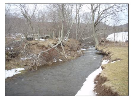
undercut trees were removed to avoid future stream problems. Live fascines, willow stakes and rock riprap were also used to stabilize the stream banks.
